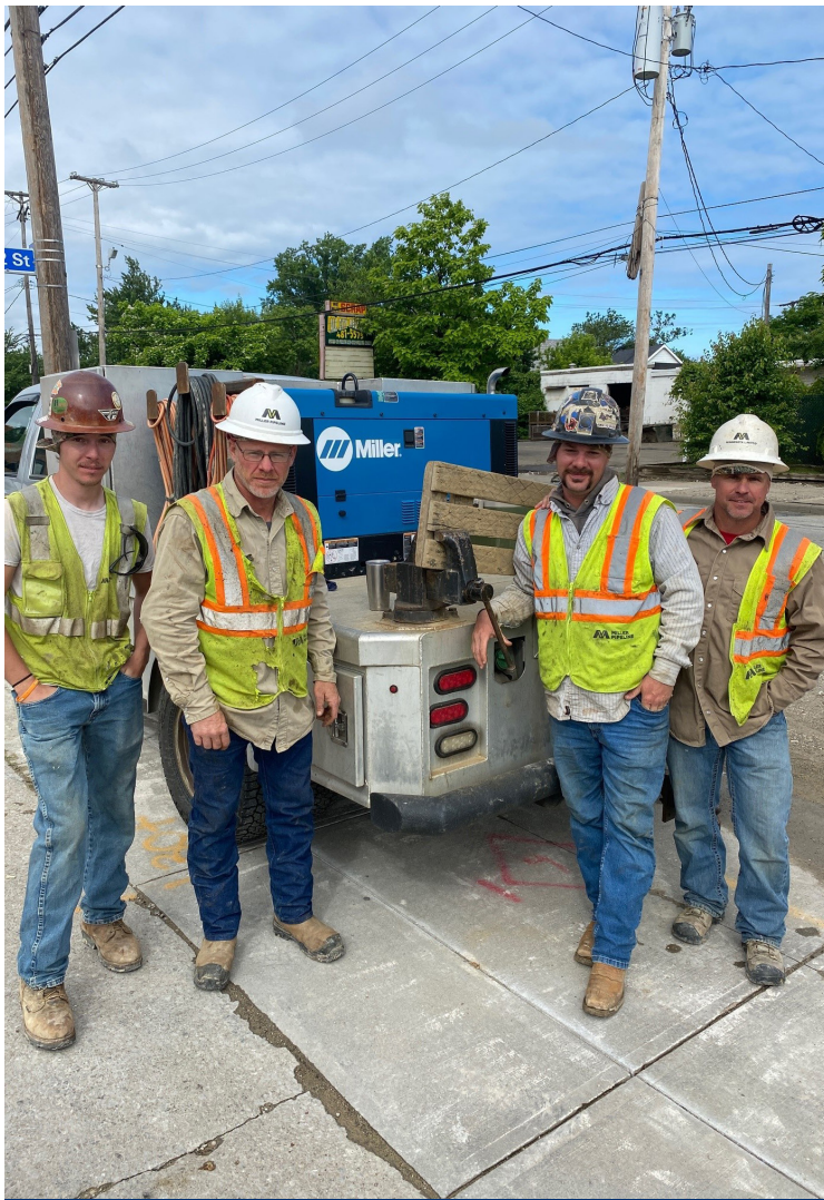
Miller Pipeline, LLC in Cleveland, OH
