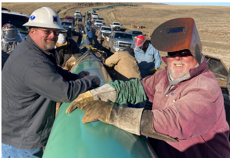
Michels Pipeline, Inc. in Watford City, ND
