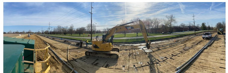
InfraSource Construction, LLC in Blue Ash, OH Submitted By: Bobby Russell
