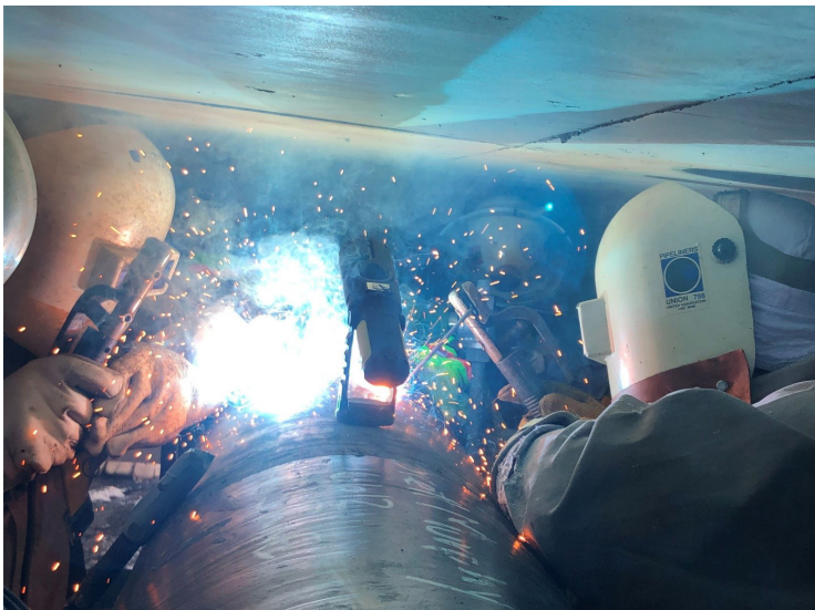
Route 147 bridge job for Columbia Gas of Massachusetts in Springfield, MA.
